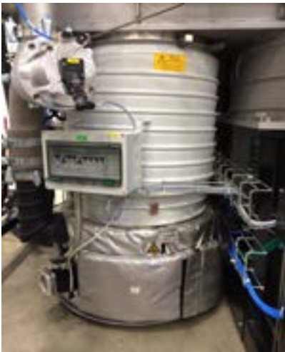
Diffusion pump and insulation.
